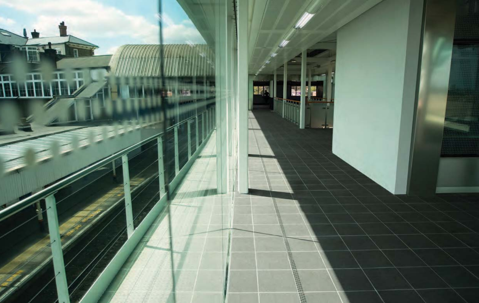
Pictured above: Gritstone Aggregate Dark Grey 300 x 300 x 9mm DW-GADGR3030 - Clapham Junction Railway Station, June 2011
